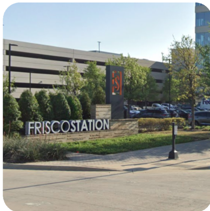
MAIN ENTRANCE TO PARKING/BUILDING
